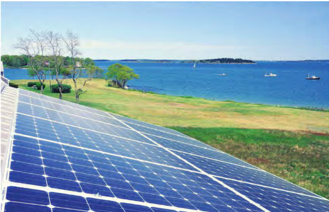
PHOTO COURTESY OF: REVISION ENERGY
